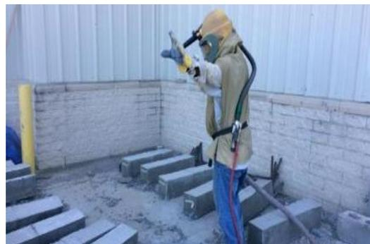
**Figure 4.** Sand Blasting of Beams
