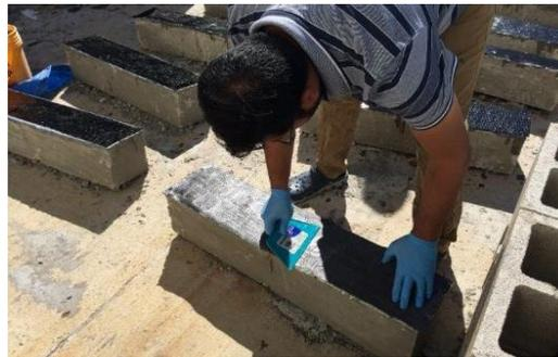
**Figure 3.** Application of CFRP laminate
